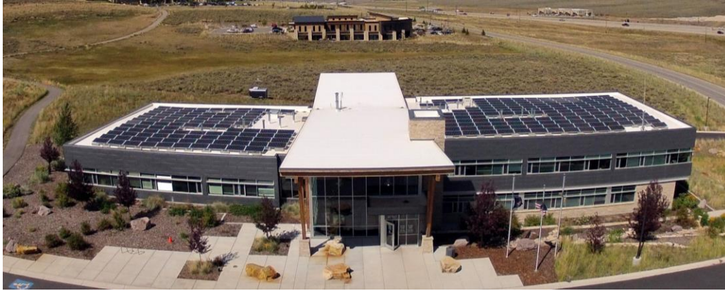
Rooftop solar on government facilities
